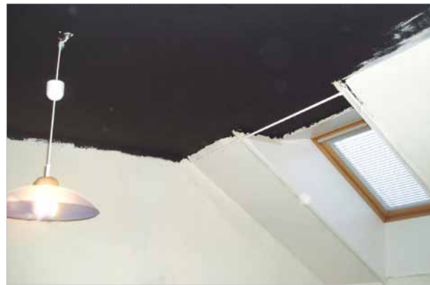
2) Application of HF shielding paint.
